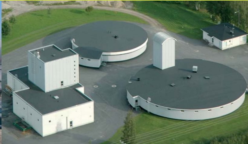
Municipal wastewater treatment plant in Kurikka, Finland
